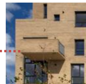
Projecting balcony with a brick front
