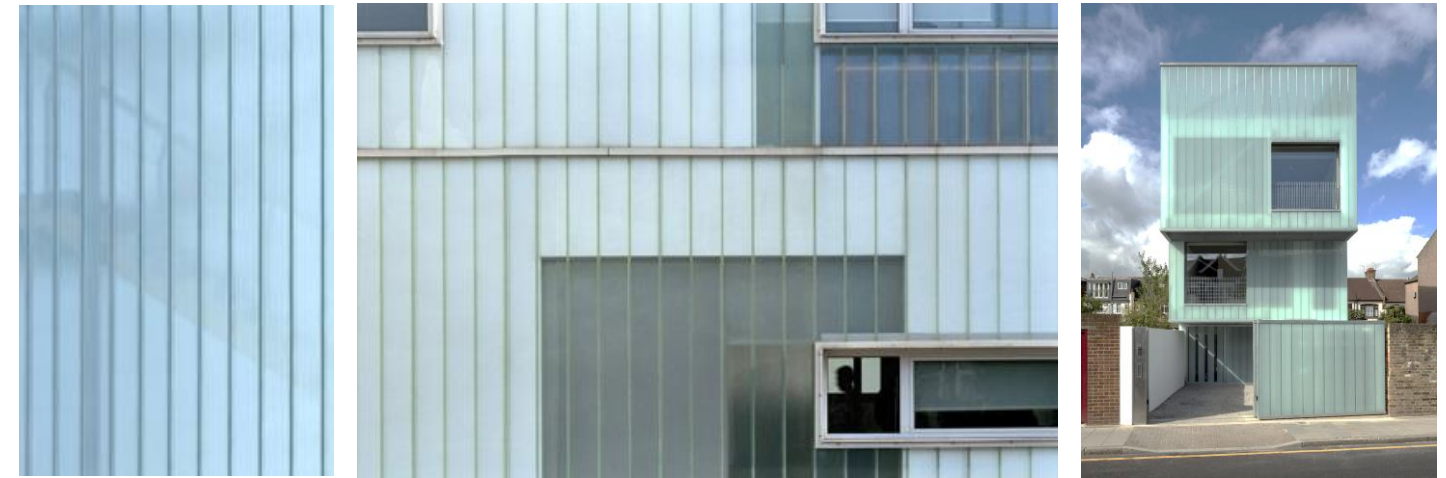
Examples of Reglit glass channels as elevation treatment
