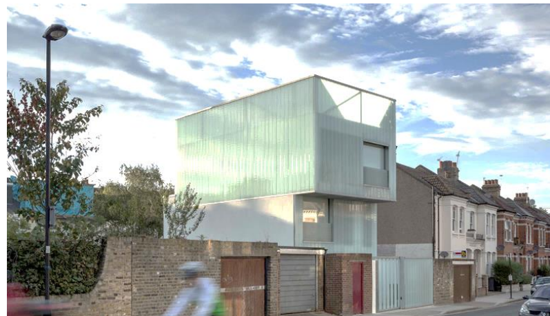
Example of glass channels used as external wall
