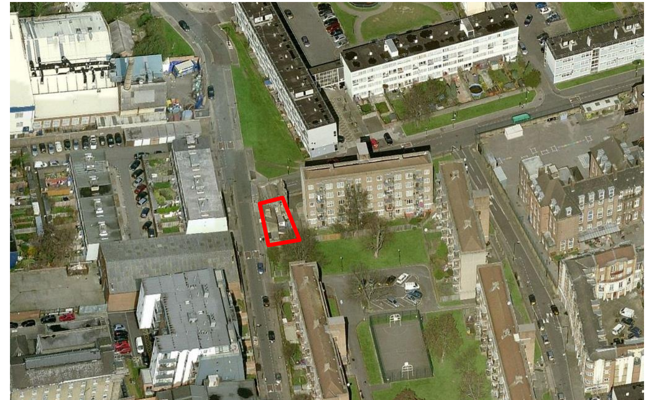
The development site seen from south
